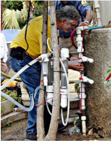
Mike Oliver, a Texas Baptist Men Volunteer from First Baptist Church in Plano, works on the water purification system for an orphanage outside Port-Au-Prince.
